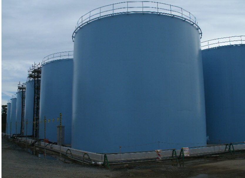
Welded type of tanks
