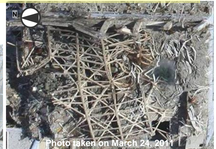
Before large debris removal
