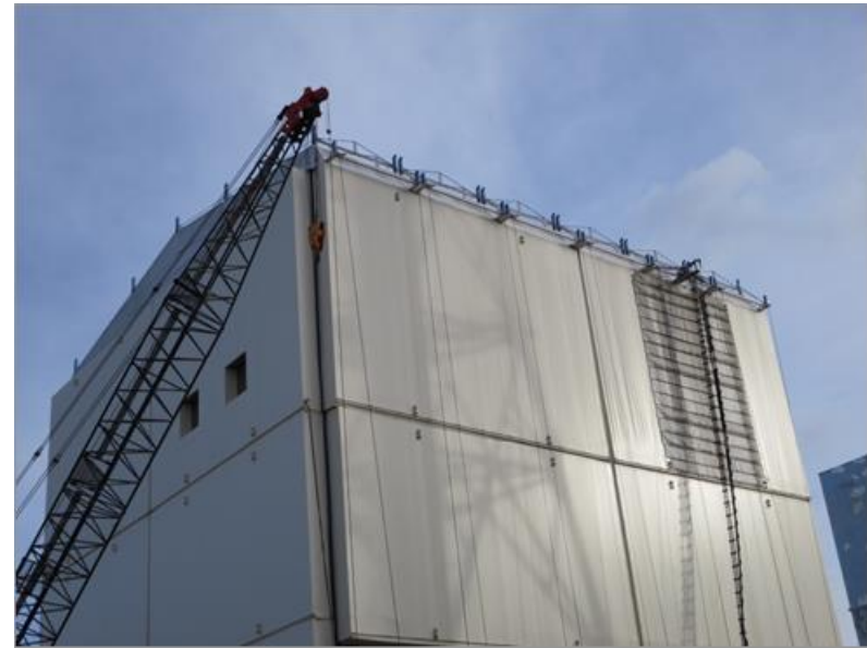
Completion of building cover structure Present
