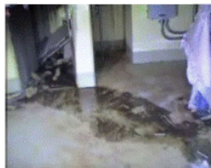
Water flow reduction confirmed (on Jan. 21)
