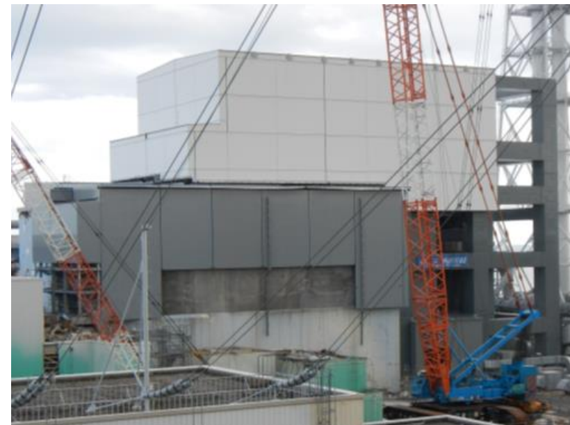
Fuel Removal Cover Structure Present
