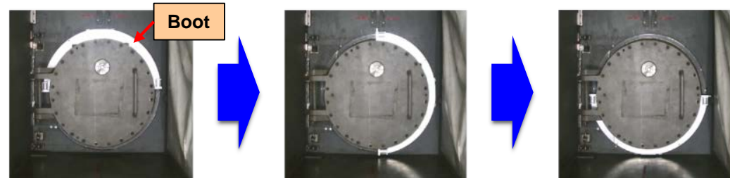
Steps for installing the lower boot
