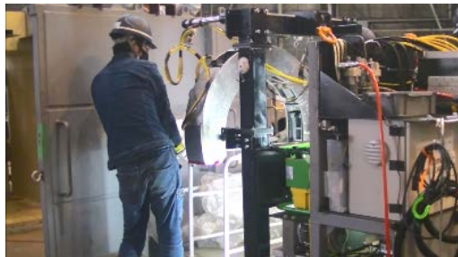
Polishing the penetration (polishing equipment being installed)
