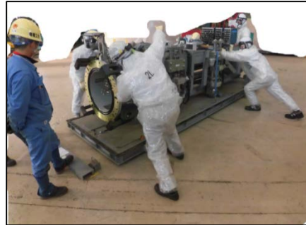
Status of carrying-in of the equipment
