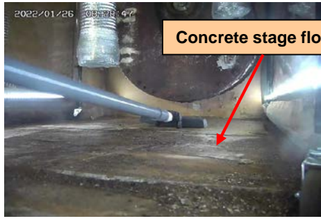
Cleaning after removing the roughness of the floor
