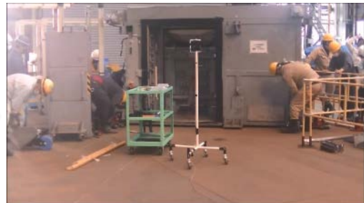
Setting up the hatch isolation room (being positioned)
