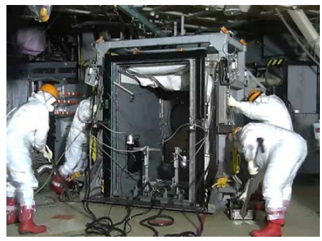
Work of installing the isolation room inside the stage
