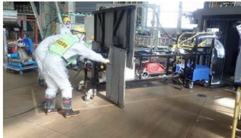
Installing the boot (Boot transportation equipment (being installed))
