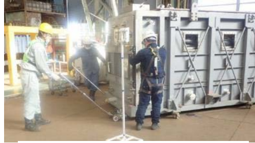
Setting up the robot carry-in chamber (being transported)
