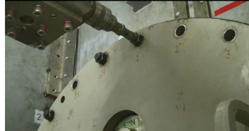
Removing the nuts and bolts of the penetration hatch
