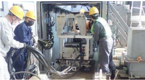
Installing the hatch opening equipment (being carried-in)
