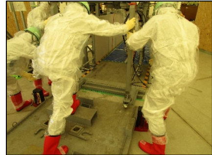
Carrying-in of the lid for preventing spread of contamination
