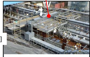
d. Cable duct installation [1]
