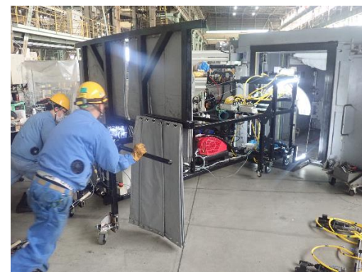
Mockup of the boot transportation equipment installation
