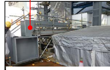
e. Cable duct installation [2]
