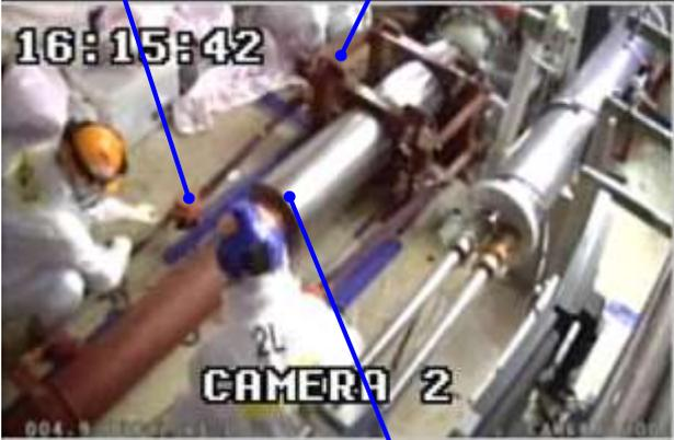
Jig for pushing in the guide pipe
