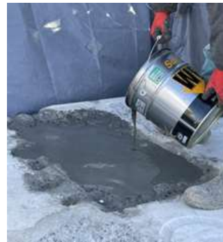
While filling non-shrink mortar
