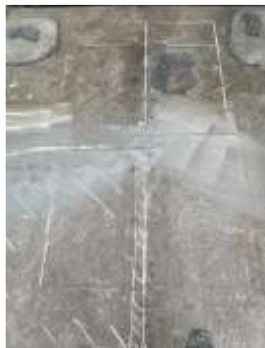
Before shaving the floor surface
