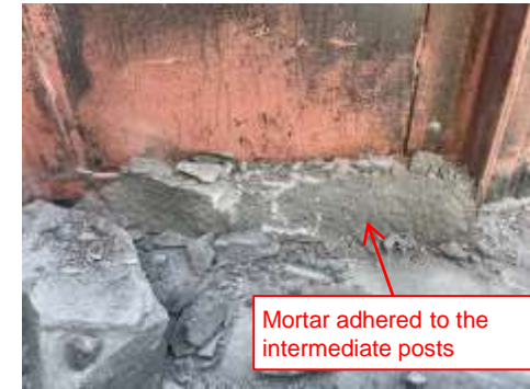
After completing disassembly of the side of the test piece
