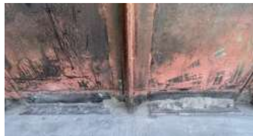
Mortar removal completed
