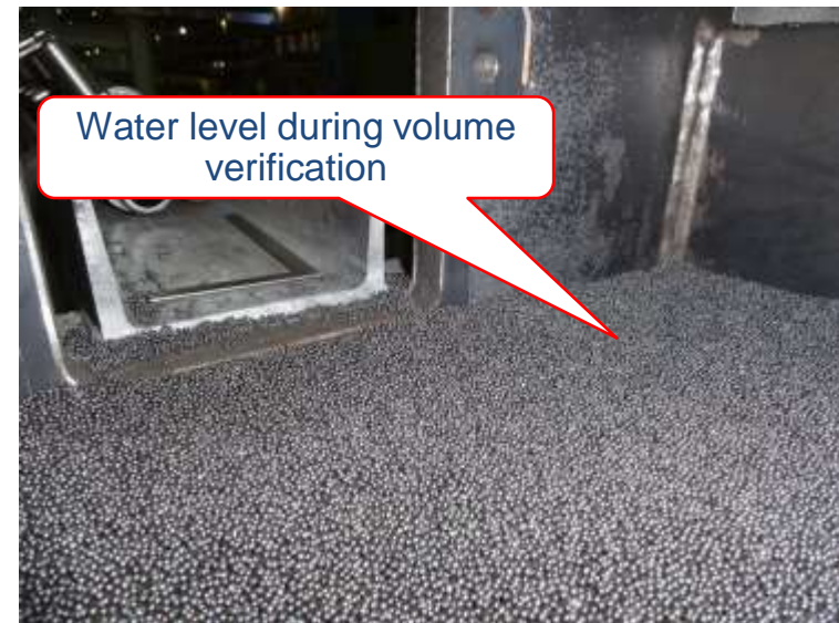
Filling status (Ceiling cell / 500m width)
