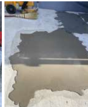
Filling completed (Right after filling)
