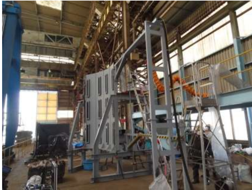
Complete view of the equipment
