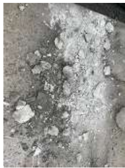
After shaving the floor surface (Before removing the disassembled piece)
