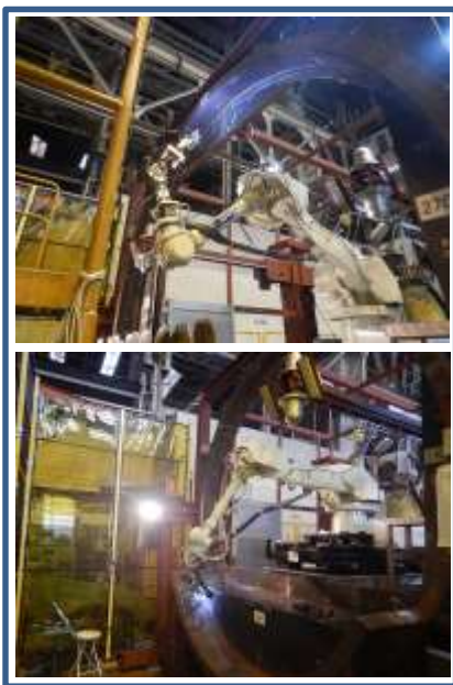
Status of remote welding using the manipulator
