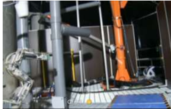
Status of the element test (Unit 2 PCV first floor)
