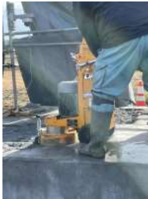
Smoothening work using a polisher
