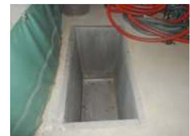
Pit for the element tests
