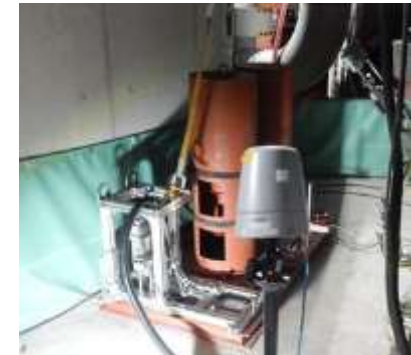
Status of the element test (Unit 2 PCV basement floor)
