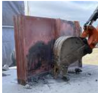
Mortar removal using a bucket
