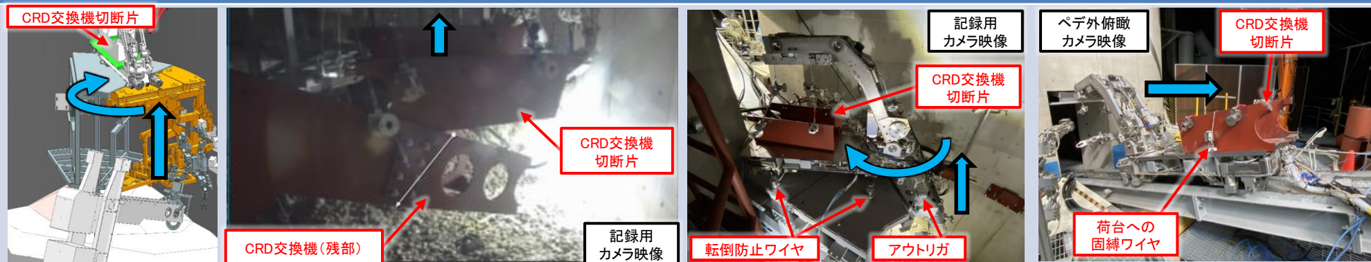
(c) CRD交換機切断片搬出
