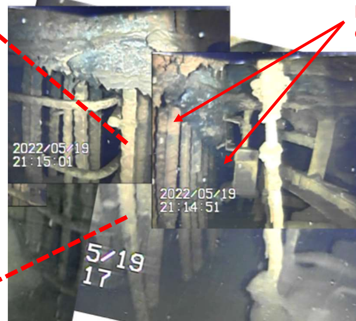
Photo 2: Concrete remains seen from the pedestal opening
