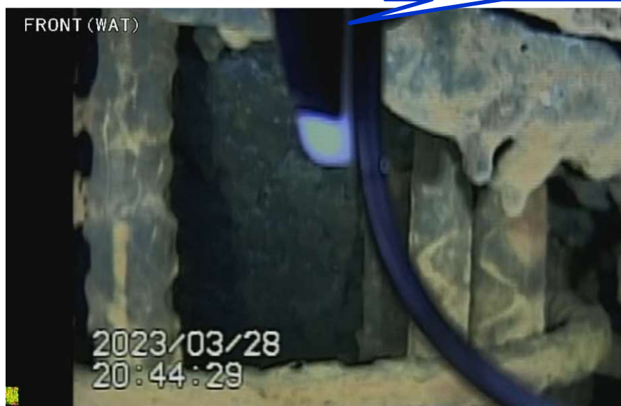
Photo 1: Concrete remains seen from the pedestal opening
