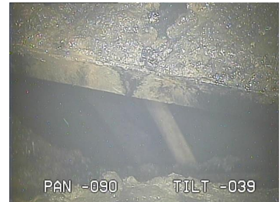
Gap between platform and CDR rail
