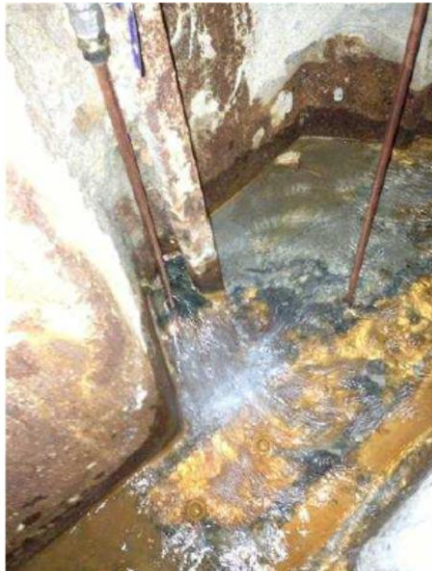
Before: (3 Lt / Second leak)
