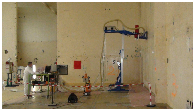
Laser decontamination system in a nuclear facility in CEA/Cadarache - France
