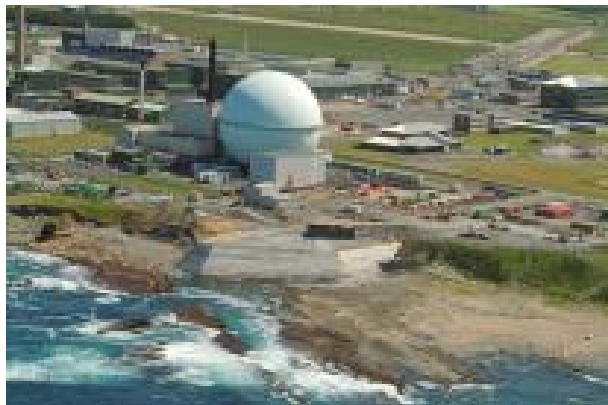
The working concrete platform built around the top of the shaft is shown above.
