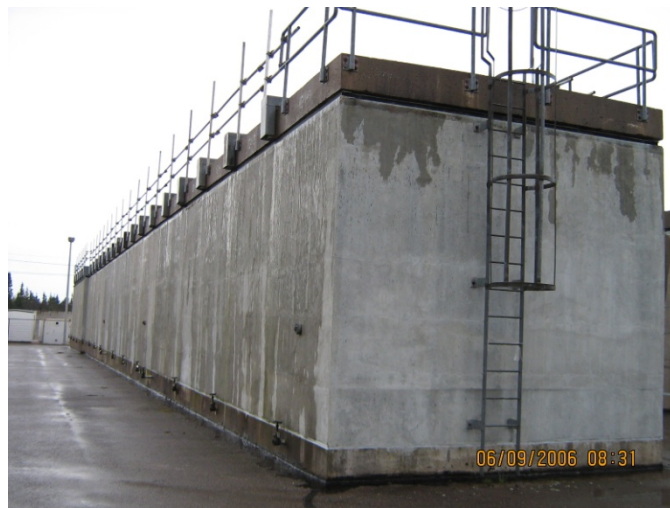
Storage Vaults for Low-Level Radioactive Waste
