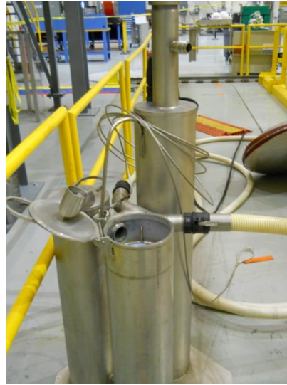
Tri-Nuc Housings- single, double, or quadruple depending on flow rate.
