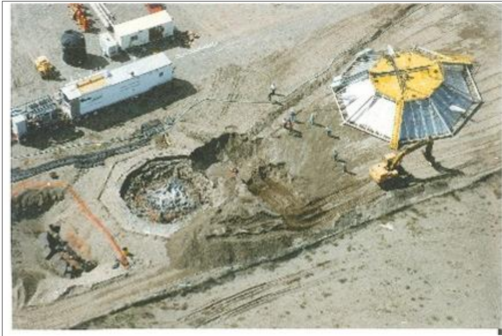
Figure 5 - Aerial view of adjacent treatment zones to create a single GeoMelt wall
