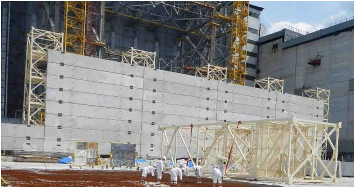
Example of tower-supported walls implemented by NOVARKA at Chernobyl (total height: 27 m)
