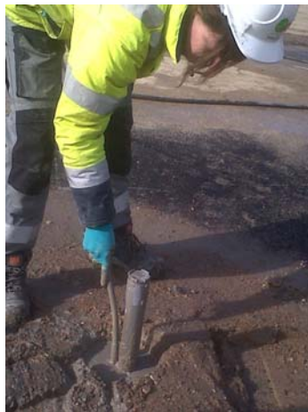
Sealing with bentonite-cement slurry
