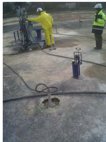
Hydraulic grouting press and equipment
