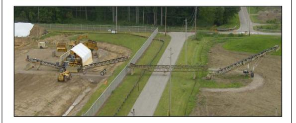
Painesville FUSRAP Remediation Project (Ohio, USA). Scanned >47,000 tons of soil and achieved a volume reduction for disposal of 35%. Less than 2% of the impacted soil volume processed required disposal as radioactive waste, saving the customer more than \$10 Million Dollars in project cost associated with the packaging, transportation, and disposal of radiologically contaminated waste.
