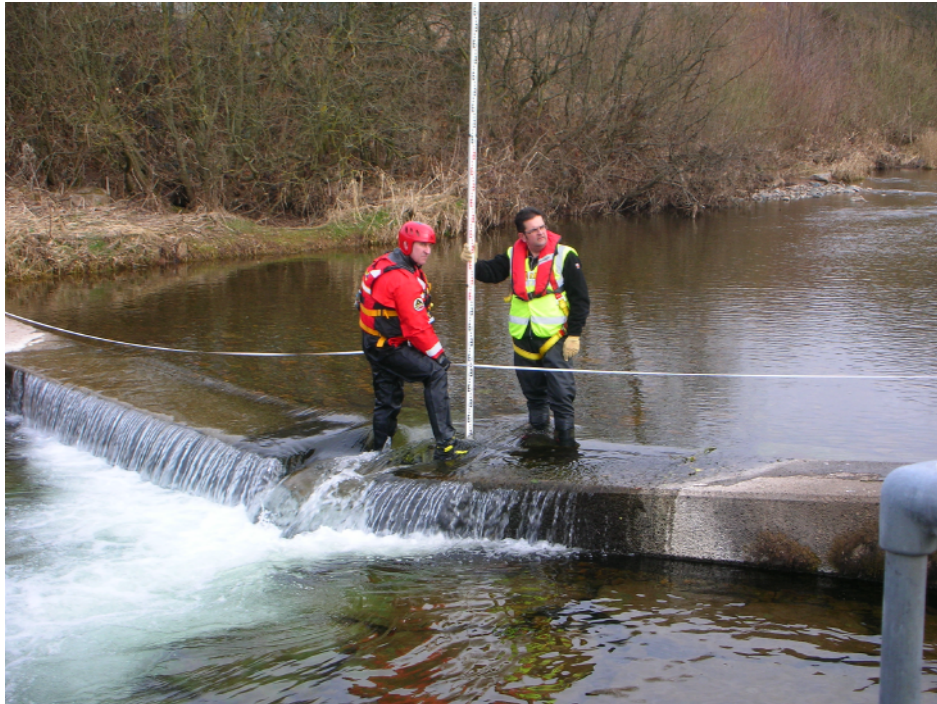
Surveying a weir during the installation of telemetry to monitor river levels
