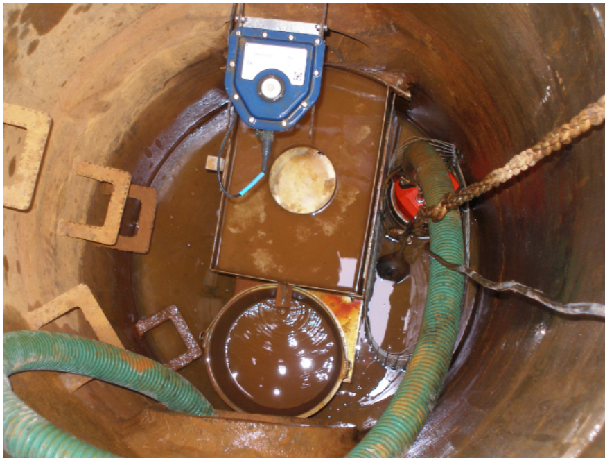
A v-notch weir positioned in a chamber to measure leachate discharge from waste trenches.
