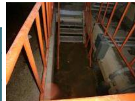
Northwest staircases area
