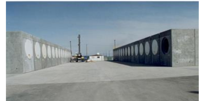
米TMI-2燃料デブリの保管システム(参考) 出展: Andrew P. Szilagyi, Three Mile Island Unit 2 Overview and Management Issues, OECD-Nuclear Energy Agency – 12th Meeting of the WPDD, France(2011)より
