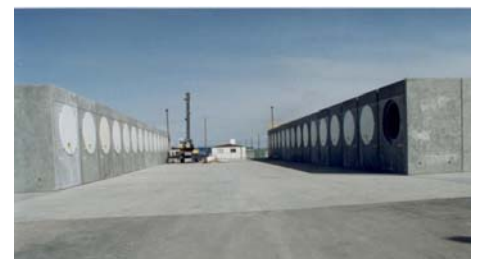
米TMI-2燃料デブリの保管システム(参考) 出展: Andrew P. Szilagyi, Three Mile Island Unit 2 Overview and Management Issues, OECD-Nuclear Energy Agency - 12th Meeting of the WPDD, France(2011)より
