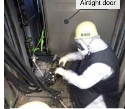
Cable disconnection task
