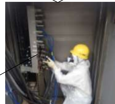
Modification of cable rack to a panel
