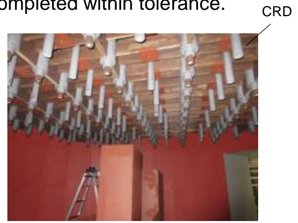
Inside the pedestal
