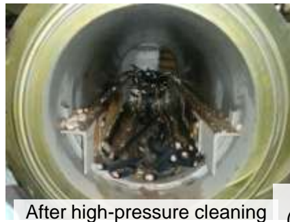
(bottom cable outside the range of passage is removed)
