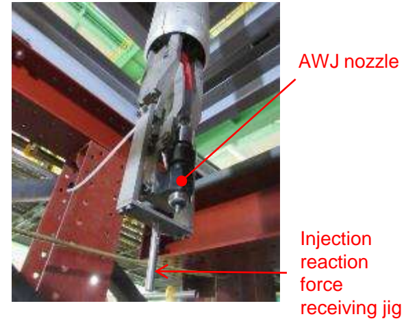
Injection reaction force receiving jig for the shroud head cutting
