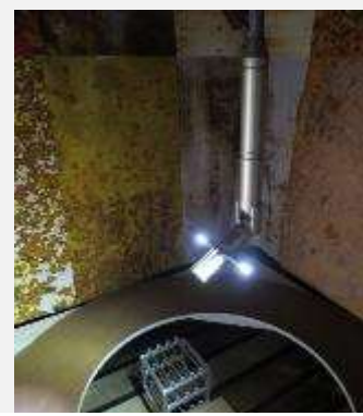
Investigation equipment B2 test
