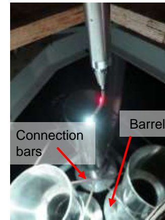
Investigation of the area under the steam dryer bottom plate (above the steam separator)
