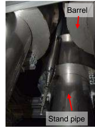
Investigation equipment passing through the area under the steam separator barrel
