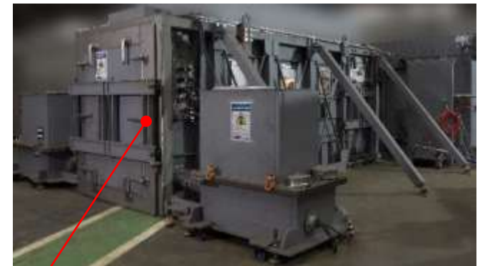
Isolation room (full view from behind)
