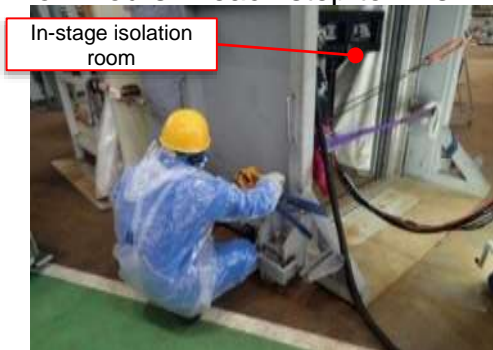
In-stage isolation room installation work
