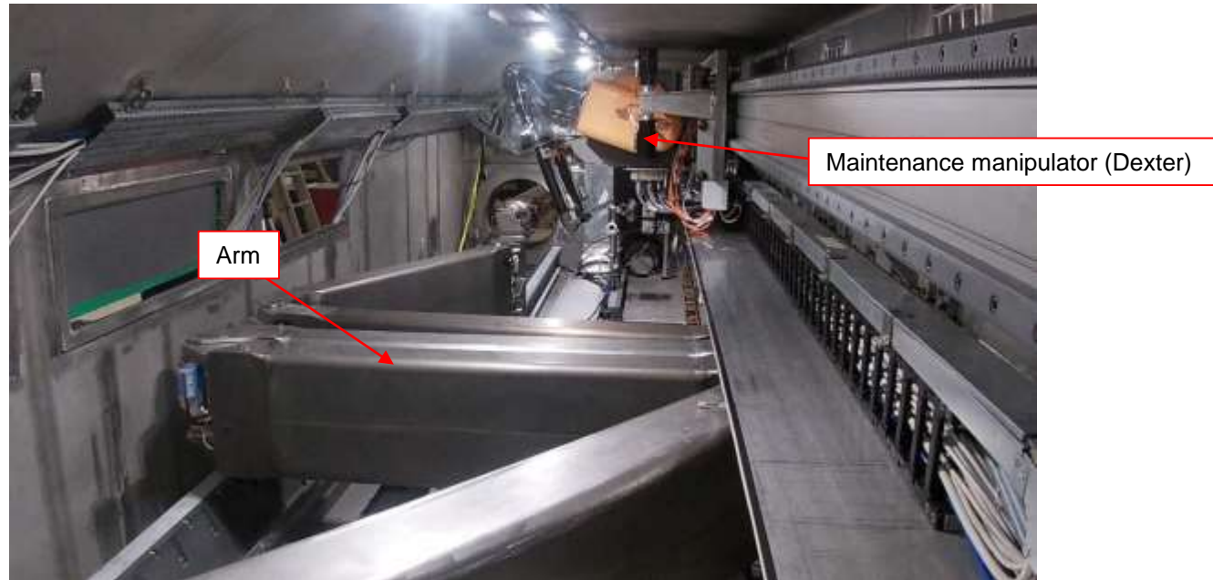
Installing equipment in the enclosure
