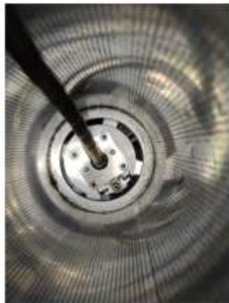
Inside the 1 st stage of the pipe after the test
