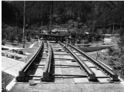
Example of a bent delivery rail
