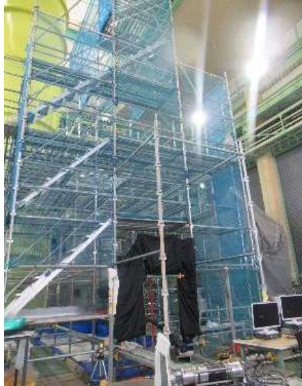
Exterior view of mockup facility 12.8 m
