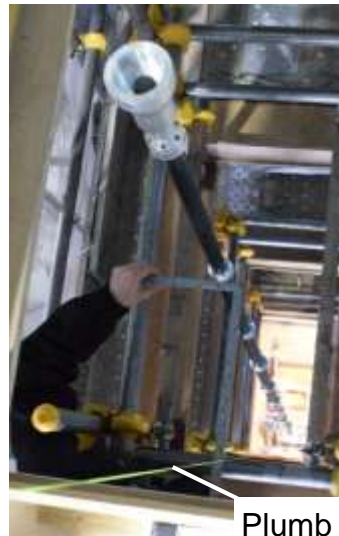
Measuring the distance from the plumb bob
