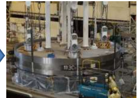
[7] Upper and lower lid lowering completion
