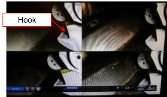
Visual image taken by the monitoring camera (Condition when lower lid does not fit)
