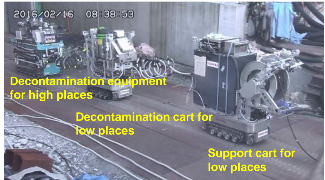
Photo of decontamination equipment moving to the Unit 3 R/B
