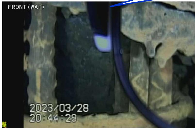
Photo 1: Concrete remains seen from the pedestal opening
