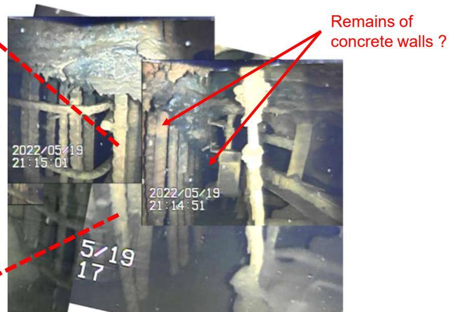
Photo 2: Concrete remains seen from the pedestal opening
