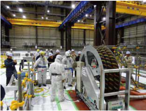
Verification test of workability to strengthen the S/C support column
