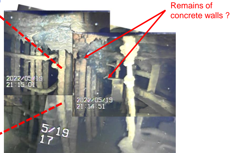
Photo 2: Concrete remains can be seen from the pedestal opening
