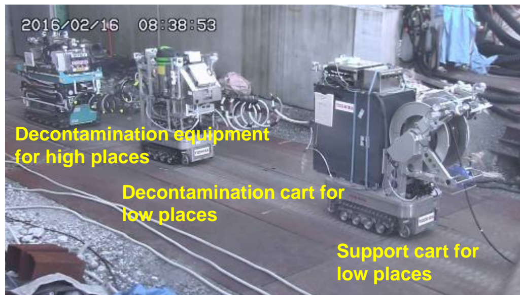
Photo of decontamination equipment moving to the Unit 3 R/B
