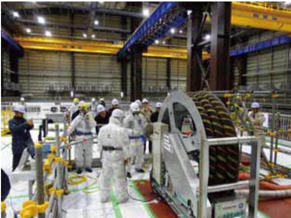
Verification test of workability to strengthen the S/C support column
